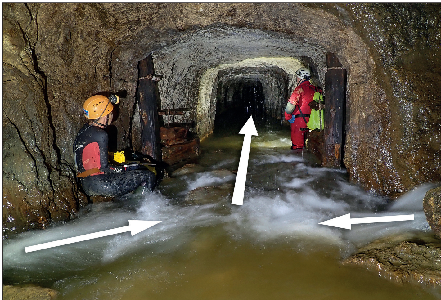
Photo 2: View facing northnortheastwards down Magpie Sough from the intersection with Townhead Vein. Water entering on the left is from Boil-up West, with Boil-up East water entering from the right.
